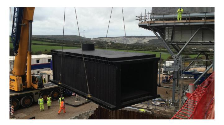
Asset expertise and Weholite technology are helping Cornwall to create a showcase wasteto-energy power plant to replace the county's shrinking landfill capacity. When complete, the new Cornwall Energy Recovery Centre (CERC) near the village of St Dennis will turn 240,000 tonnes of household waste a year into enough electricity to power 21,000 local homes.
