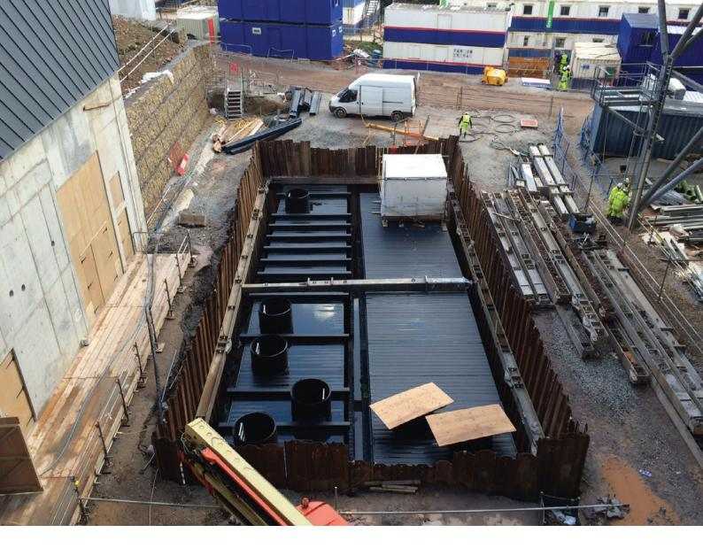
Weholite's polyethylene solutions were chosen over competitors using more traditional materials – such as concrete – due to the fact that they are quicker to deliver and install, and exceed other materials in resilience and longevity.
