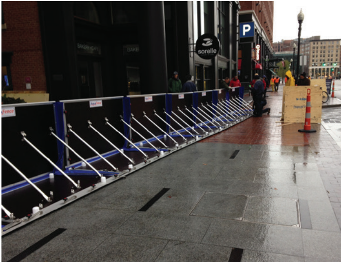
ATLANTIC WHARF, BOSTON RETROFIT EXISTING STRUCTURE IN NEWLY DECLARED FLOOD ZONE
