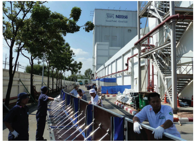
NESTLE, THAILAND FACTORY PROTECTION
