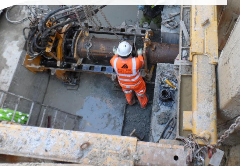
Prevailing ground conditions and the knowledge and experience of operatives regarding the use of appropriate tooling and polymers are always significant because these factors are fundamental to a successful directional drilling operation.
