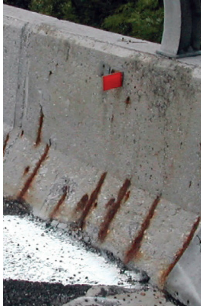
Exposed rebars due to the effect of carbonation
