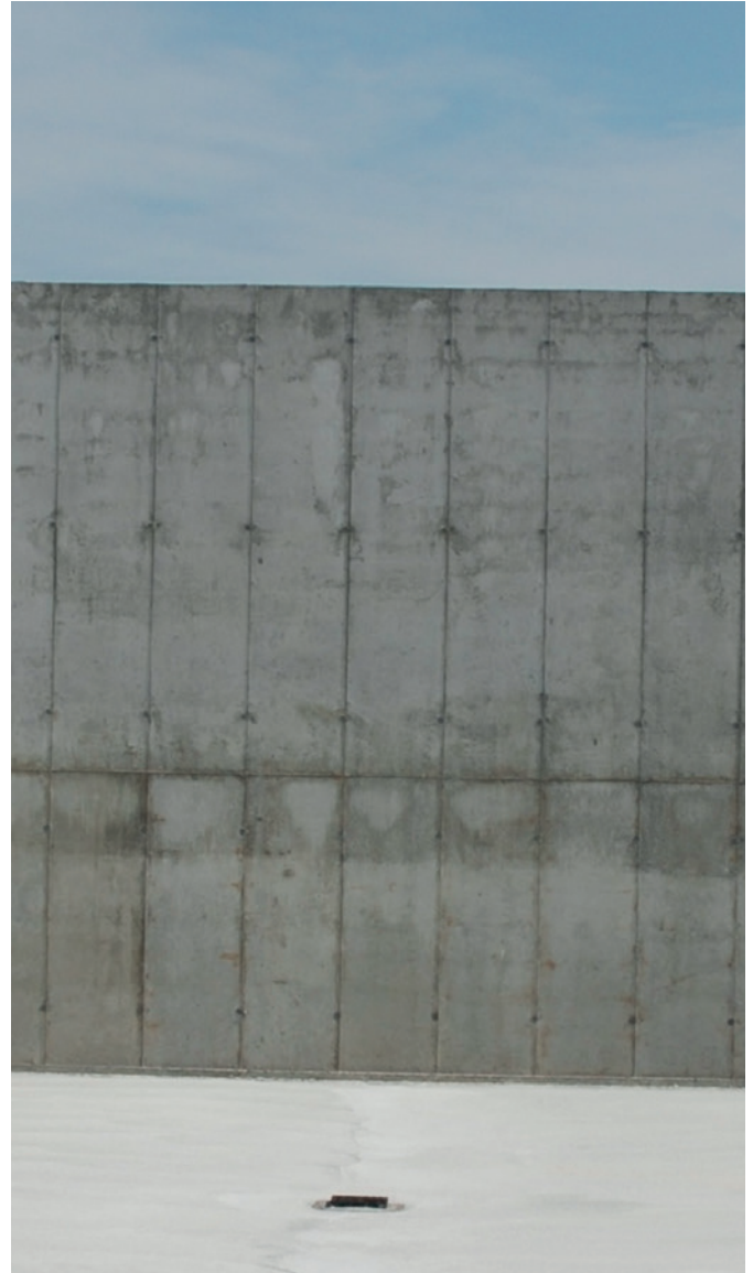
A concrete wall. As it sets, concrete diminishes in volume by 1%
