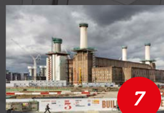
Iconic Battersea Power Station chimneys rebuilt
